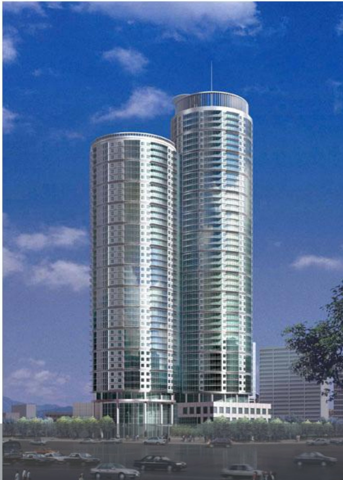
D.R. HASSAN FAIRD HOTEL AND OFFICE BUILDING- ABU DHABI
